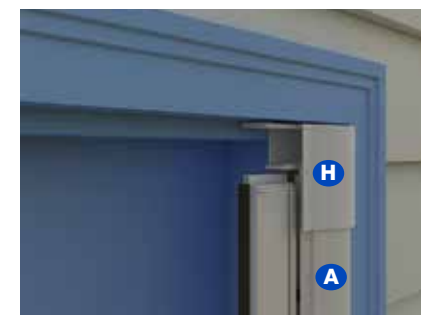
7.2 Slide the Boot Body to the Top of the Opening
